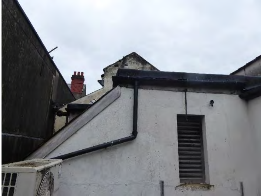
Figure 35 Profile of clerestory lighting to parallel ranges visible from roof
