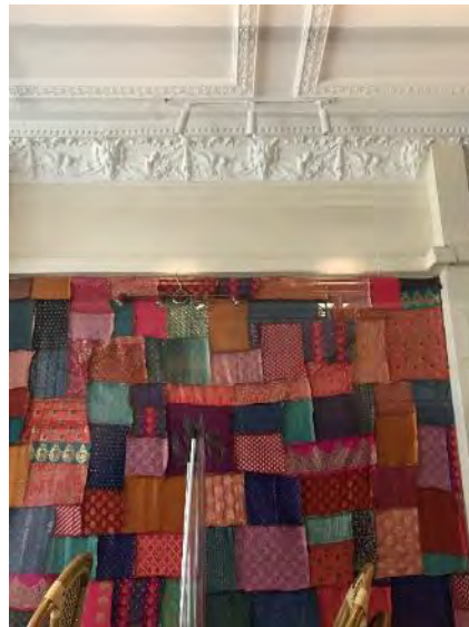
Figure 32 ceiling of No. 1
