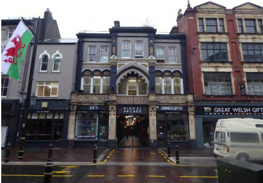
Figure 11 Entrance to High Street Arcade from High Street
