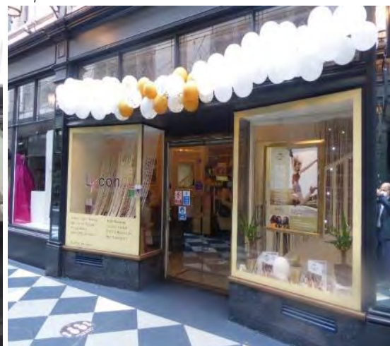
Figure 20 Splayed shopfront to No. 13
