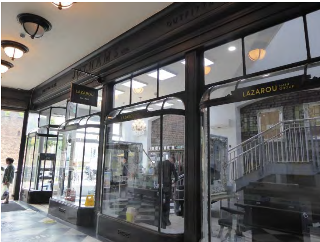
Figure 27 Former Jothams shopfront at north-east end of arcade
