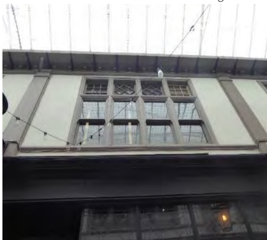
Figure 19 Typical 1 st floor window
