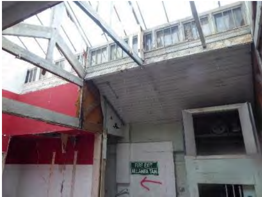
Figure 37 Boarded soffits in parallel range to south
