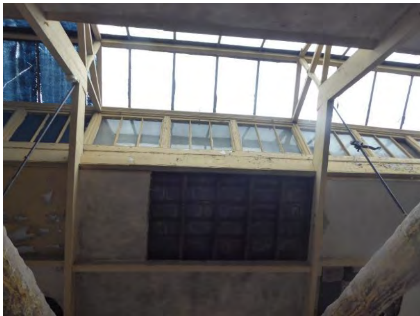
Figure 36 Clerestory lighting and timber trusses to parallel ranges behind High St Arcade
