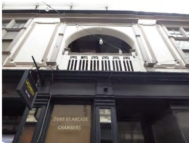
Figure 28 Duke Street Chambers 1 st floor landing
