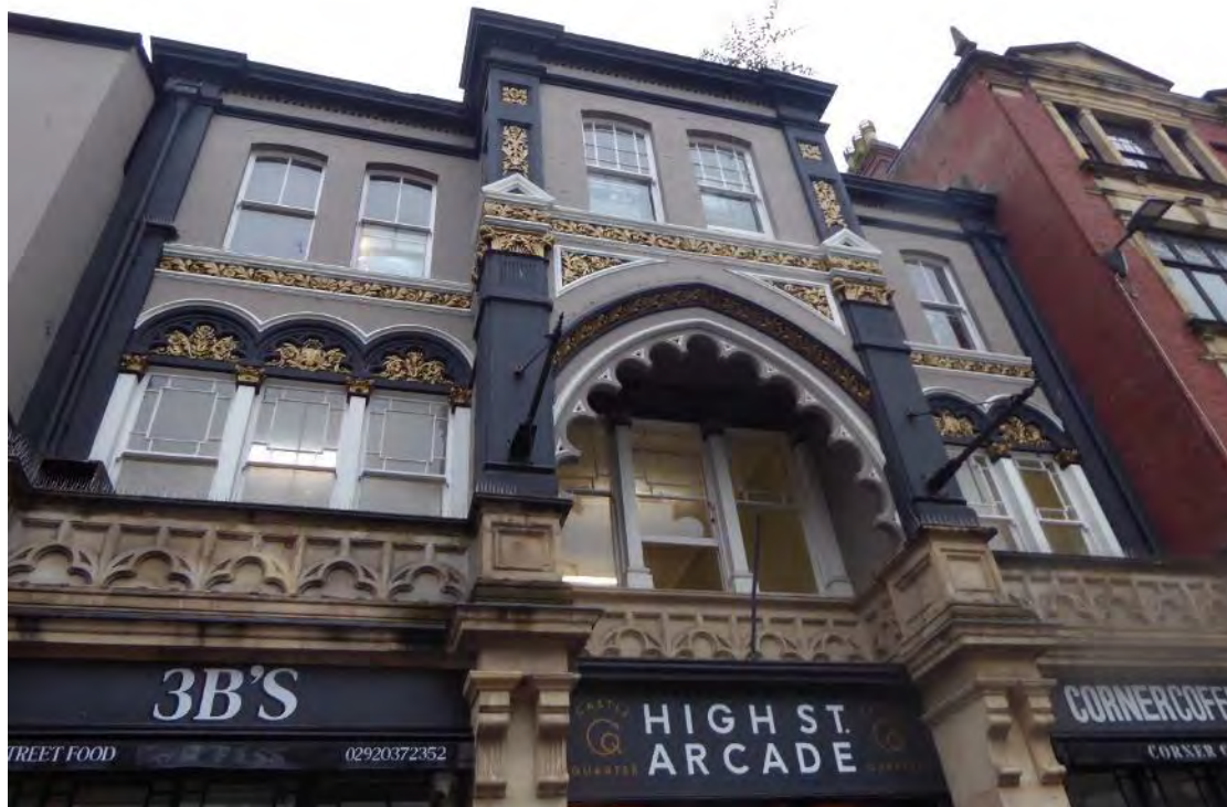
Figure 13 Upper floors of High Street Arcade frontage to High Street
