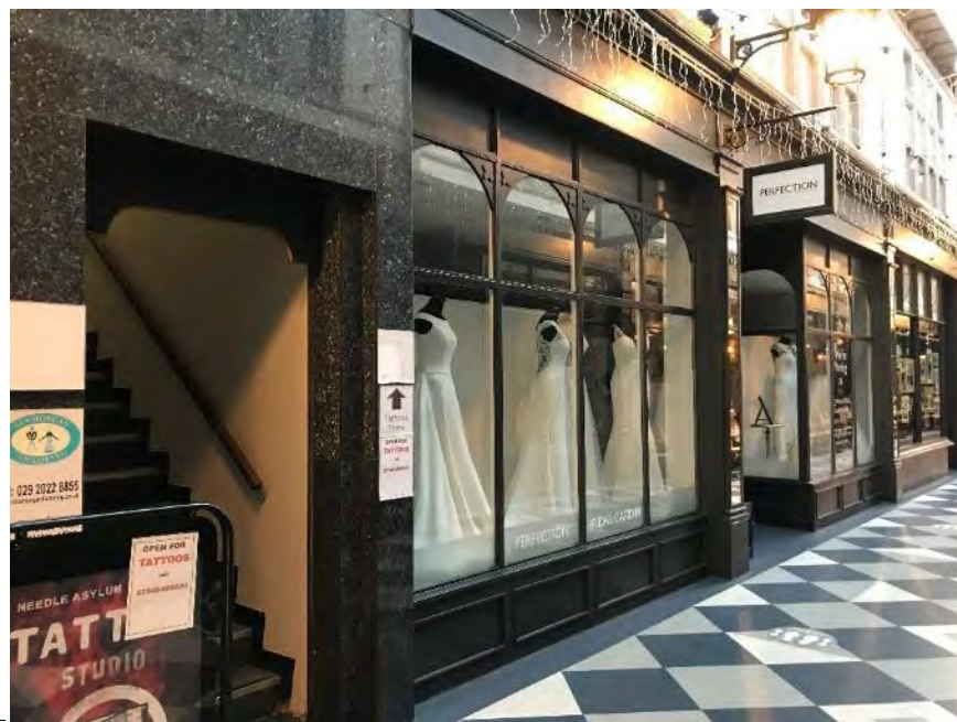
Figure 42 Shopfront to Nos 3-5 and staircase between it and No. 1
