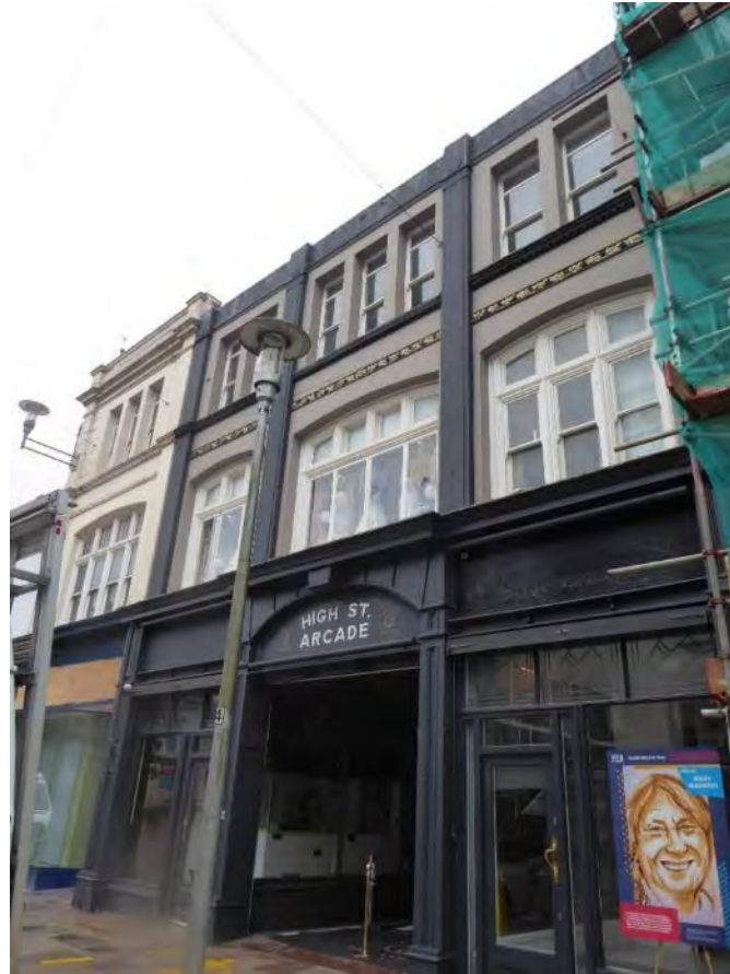
Figure 14 High Street Arcade entrance block facing St John Street
