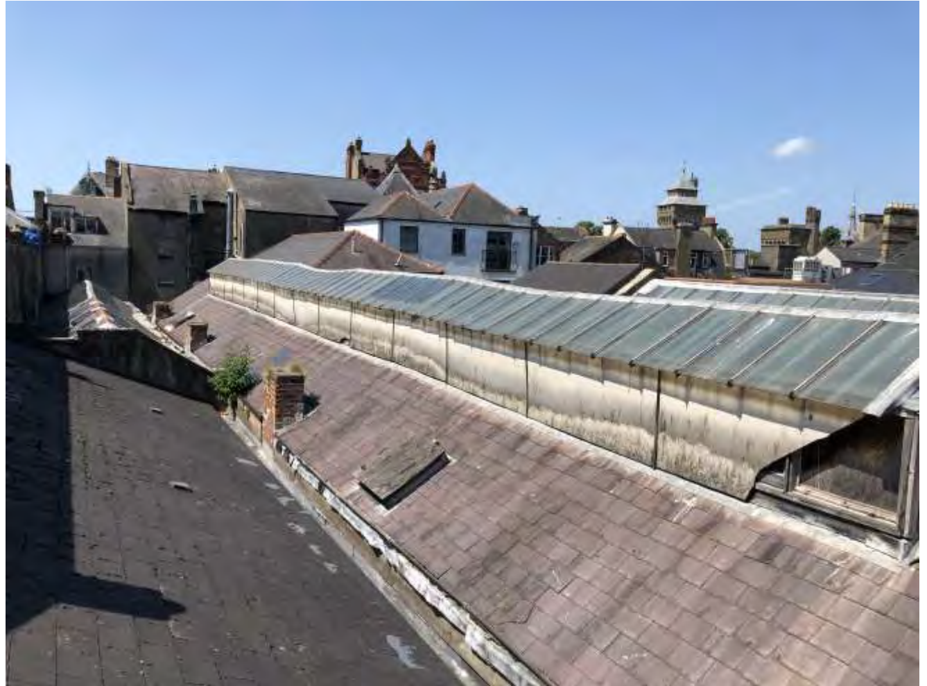
Existing Roof layout
