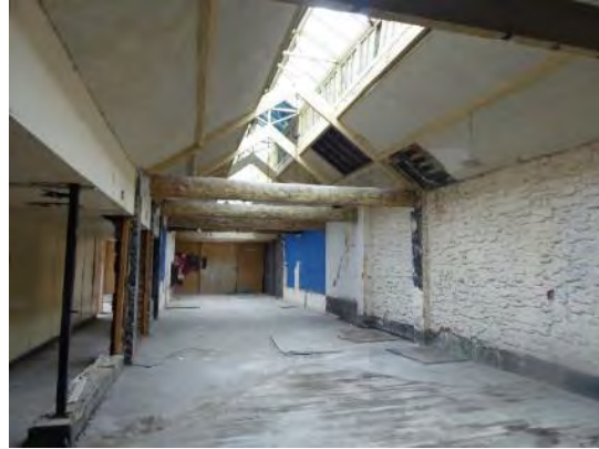
Figure 38 Parallel range to north
